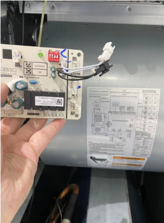
7. Install a new board, set the capacity dip-switch per the wire diagram on the unit.
