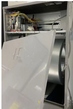
2. Remove front panel
